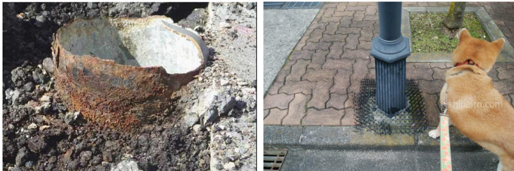
Figure 1. Left: Base of Telegraph Pole Corroded by Dog Urine (Noriyuki Suou,2021) Right: Spike Mat to Prevent Dog Urination (Arisa Shirahama,2019)
